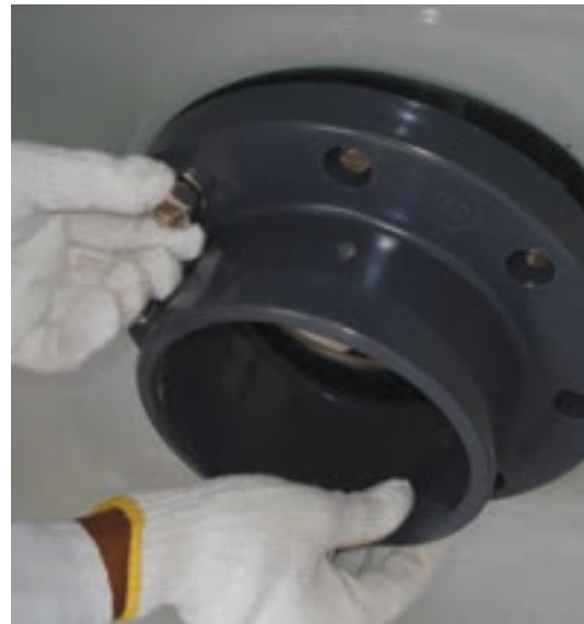
Fitting Flange with Rubber, Gasket and Rubber Capped Bolts
