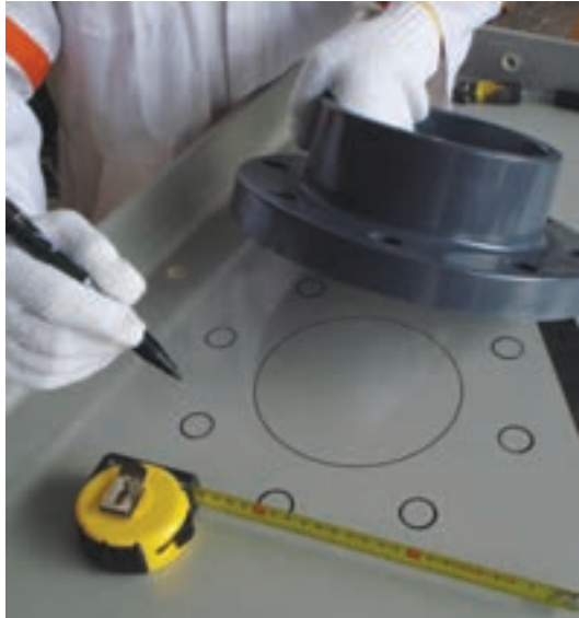
Marking Flange Hole and Bolt holes at relevant location
