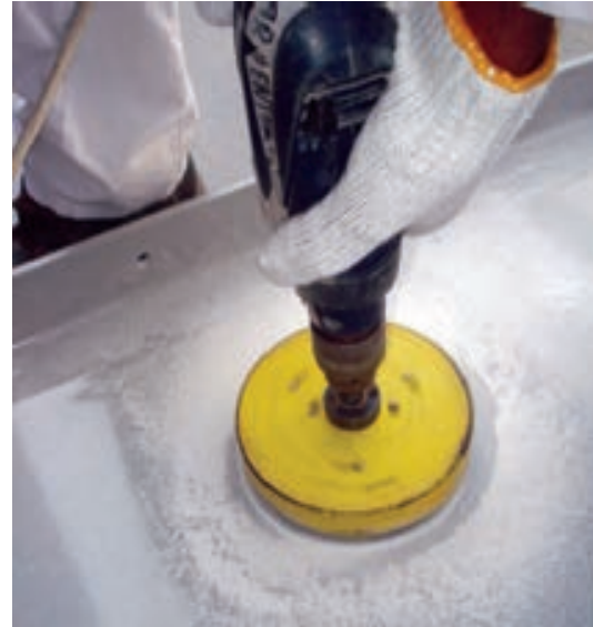
Drilling Flange hole
